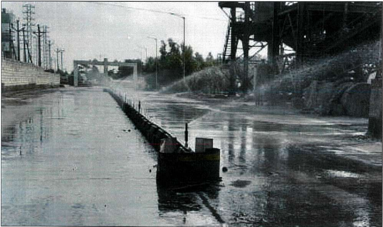
FIXED WATER SPRINKLERS ARE ARRANGED ON ROADS
