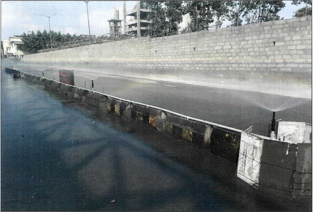
FIXED WATER SPRINKLERS ARE ARRANGED ON ROADS
