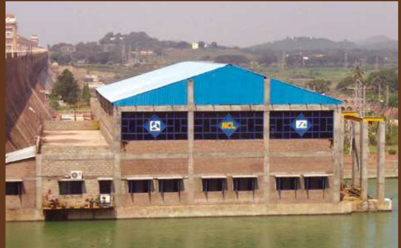
Hydel Power House at Tungabhadra Dam.
