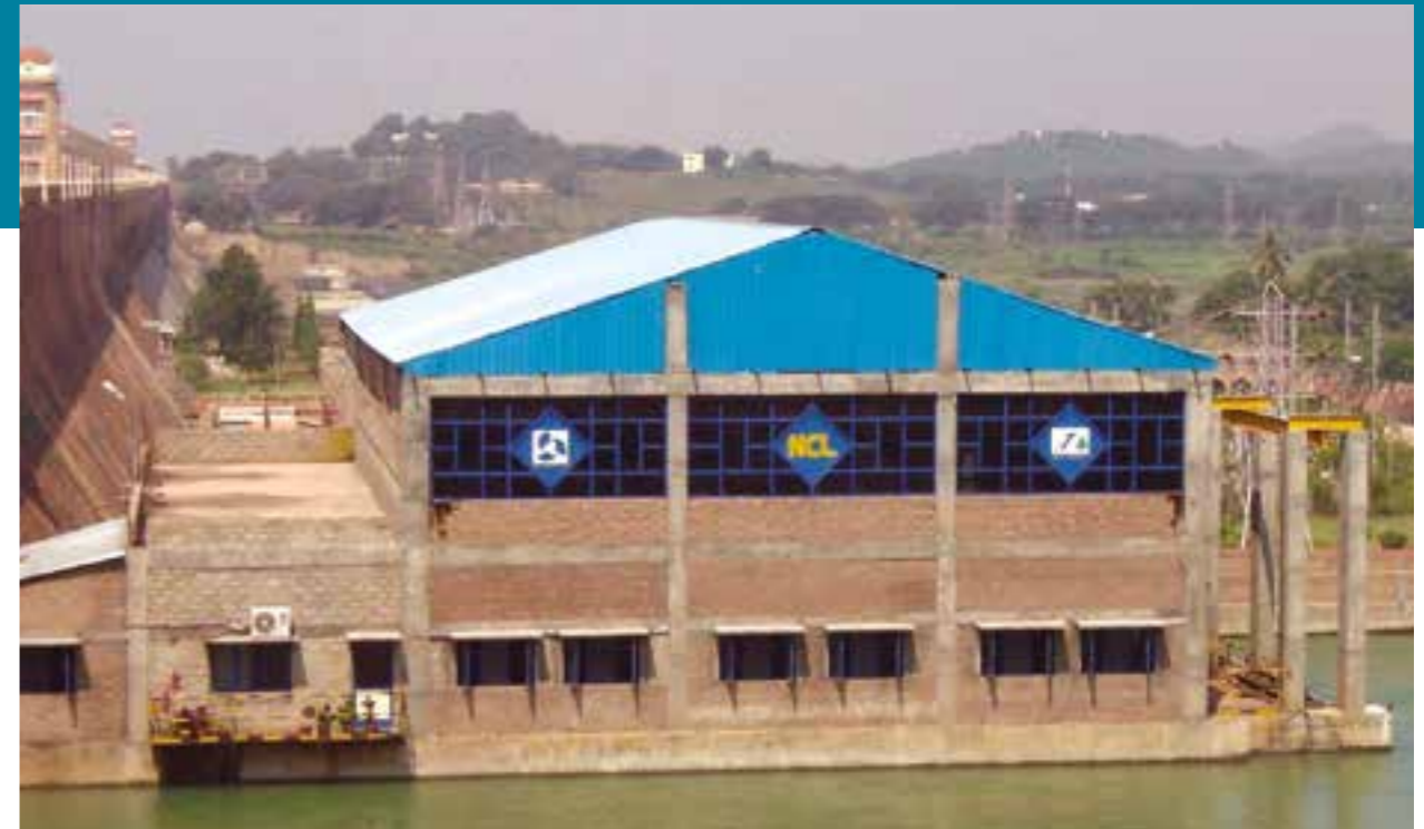
Hydel Power House at Tungabhadra Dam.
