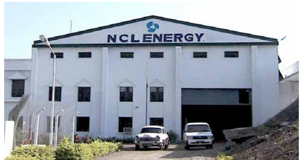
Hydel Power House at Sri Sailam Dam
