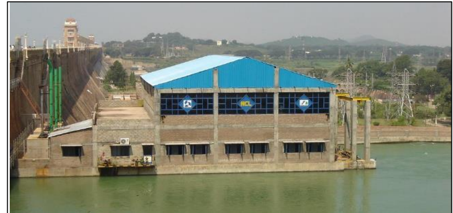
Hydel Power House at Tungabhadra Dam
