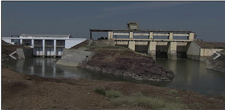
Hydel Power House at Srisailam Dam
