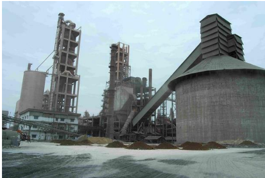
Telangana Cement Plant
