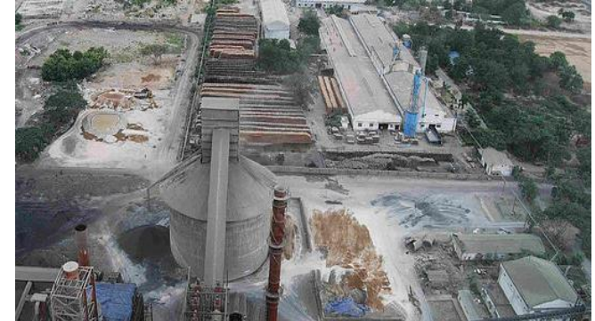
Telangana Cement Plant
