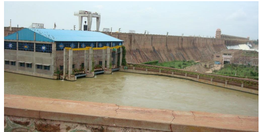
Hydel Power House at Tungabhadra Dam
