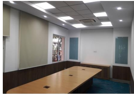
Wall Cladding & False Ceiling
